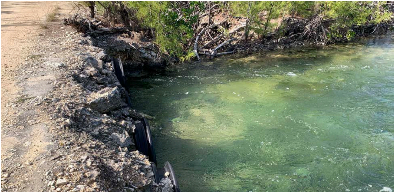
Figure 12. Culverts were installed to restore natural water flow to the mangroves previously impacted by the construction of a road accessing the coast near Broad Creek in Abaco. Credit: Lianna Burrows.
