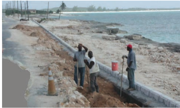
Figure 19. This road on the west coast of San Salvador has led to the destruction of the beach, once like the shore in the background. This has led to road damage and now the construction of a sea wall to protect the road. Credit: Neil Sealey.
