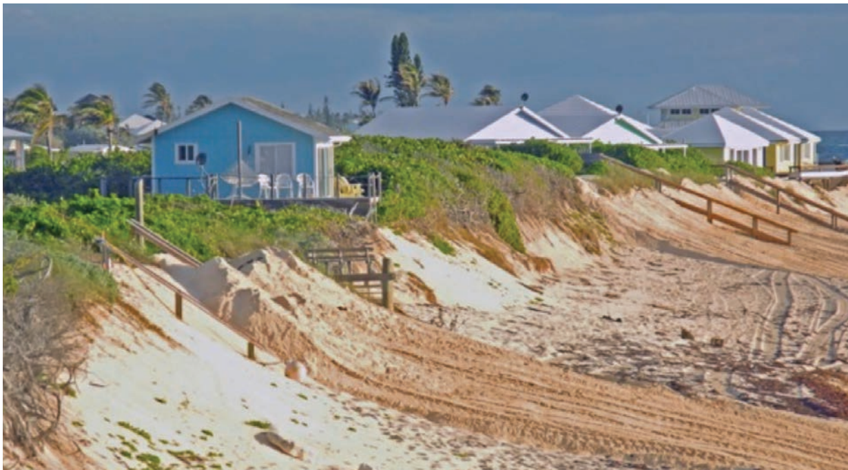
Figure 21. Sand scraping on Elbow Cay, Abaco, after Hurricane Sandy. Bulldozers or bobcats pushed foreshore sand up the beach to replace sand eroded from the dune face. Ideally houses should not be built on sand dunes. Credit: Neil Sealey.
