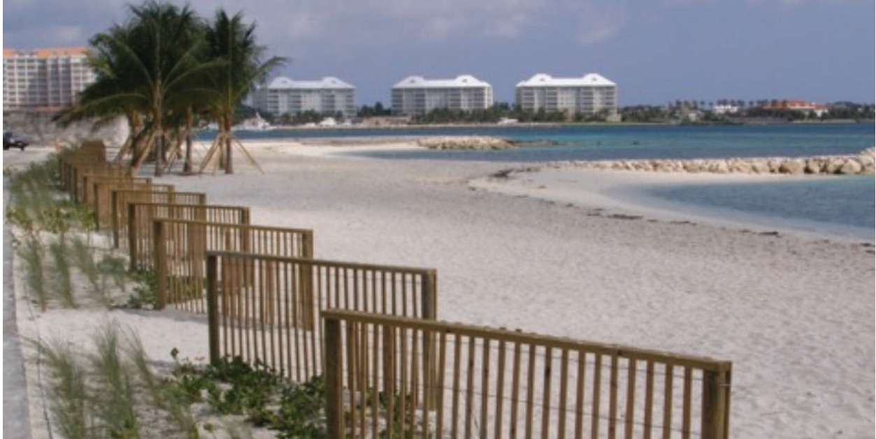
Figure 17. Sand fencing and vegetation planting on Montagu Beach, Nassau. The beach has also been reclaimed with sand from Exuma, and mushroom groynes (background) constructed to preserve the new beach. Credit: Neil Sealey.
