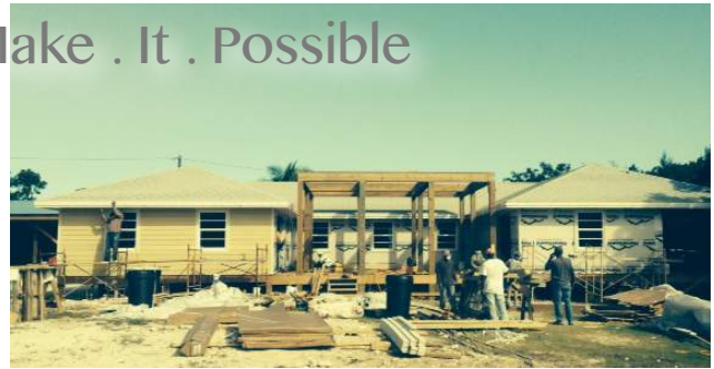
Construction progress as of (Jan. 21)
