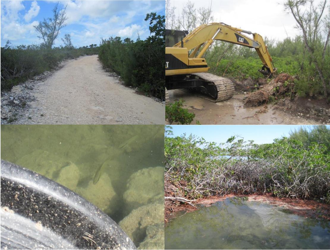
Figure 2. The road to Camp Abaco blocked 28 acres of wetland area (top left). The first step in the restoration was to remove the road, put the culverts in place, and then re-build the road. This step of the project was completed with an excavator (top right). Rocks were placed around the mouth of the culverts to stabilize the road and provide habitat for small snapper (bottom left). Areas were cleared on each side of the culverts to provide for freely flowing water (bottom right).
